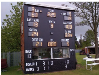
Score Hut Refurbishment
